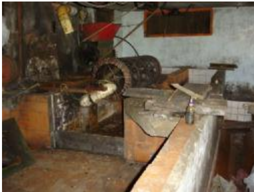
Original facilities to process the coffee based on water consumption.
